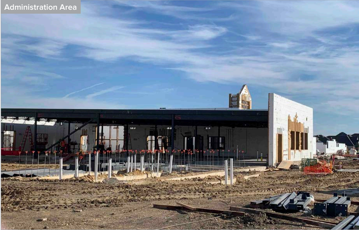
ICF Along Rear Elevation
