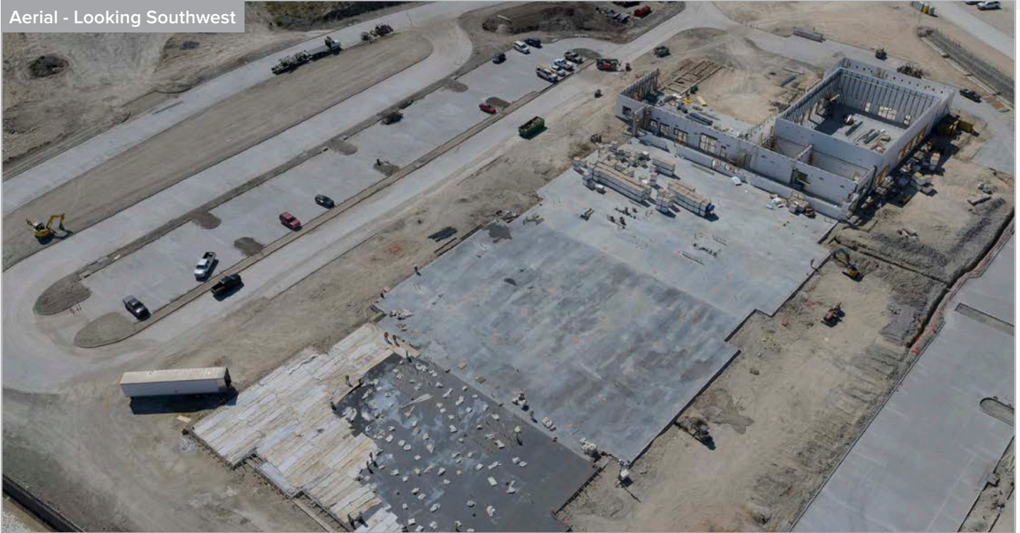
Forming of Site Retaining Wall Along Coit Road
