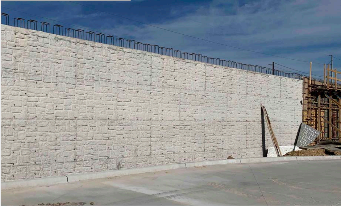
Site Retaining Wall Along Coit Road
