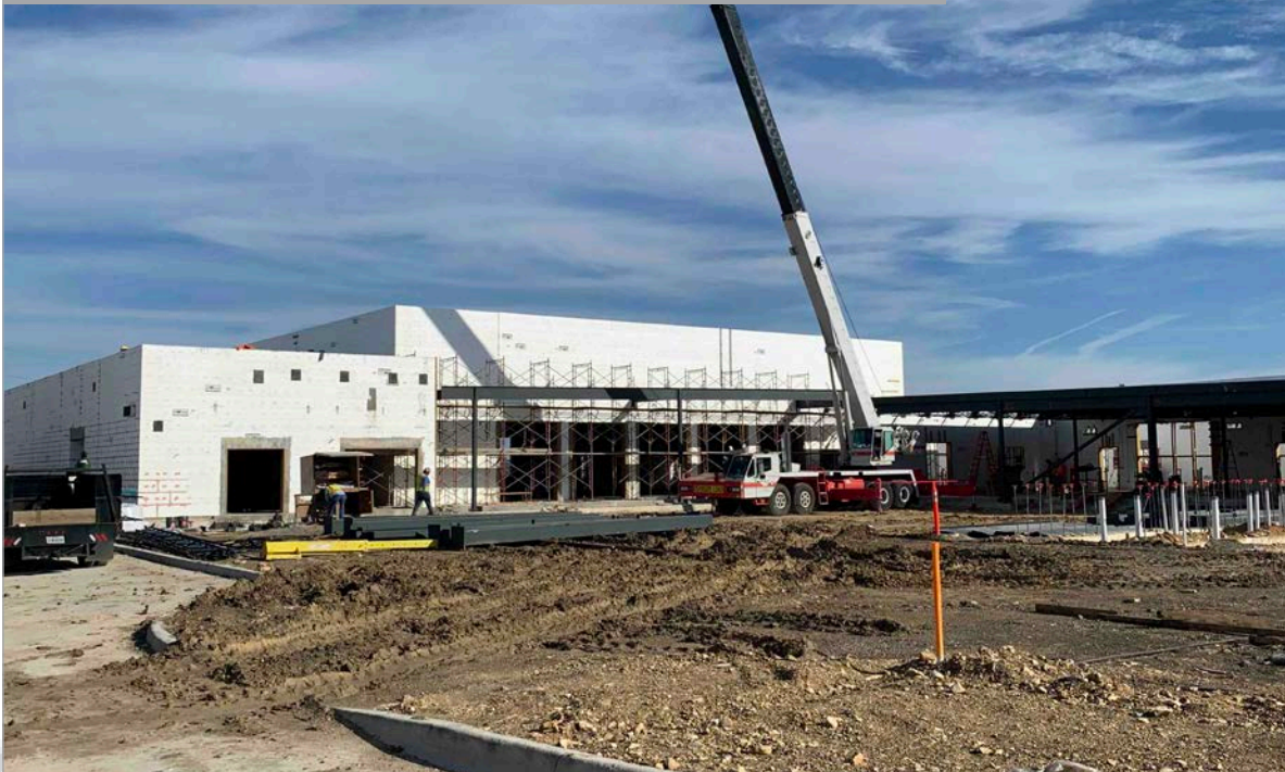
Placing Structural Steel at Secondary Corridor (Cafetorium/Gymnasium)
