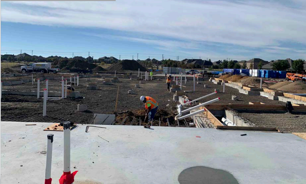
Preparing for Void Form Placement
