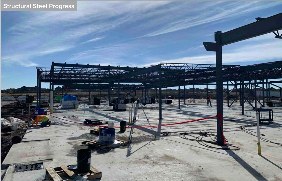
Structural Steel at Library
