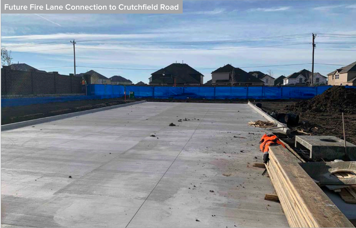
East Property Line Fire Lane
